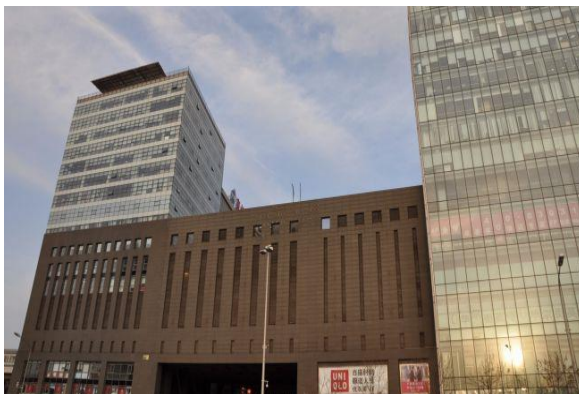
Figure 9 TESTEX Institute – Zurich (Switzerland)
